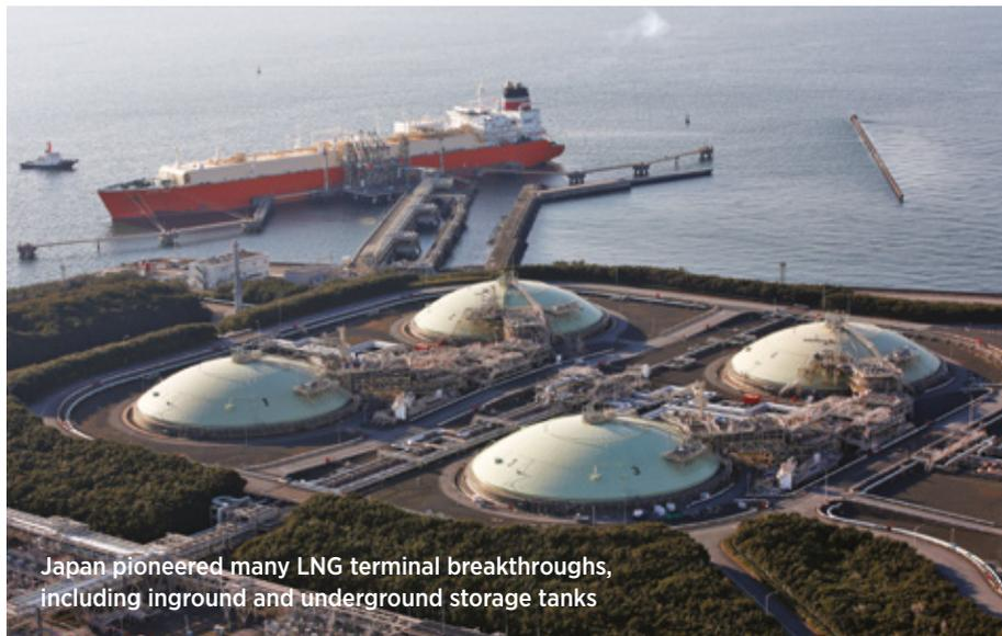
Japan pioneered many LNG terminal breakthroughs, including inground and underground storage tanks
